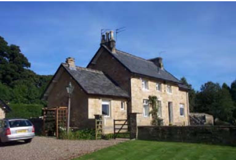
(11) Station House although un-listed is of considerable quality and provides a valuable link the village's past.
