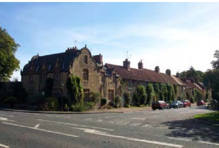
(12) 1-12 The Village a terrace of Grade II Listed Building.
