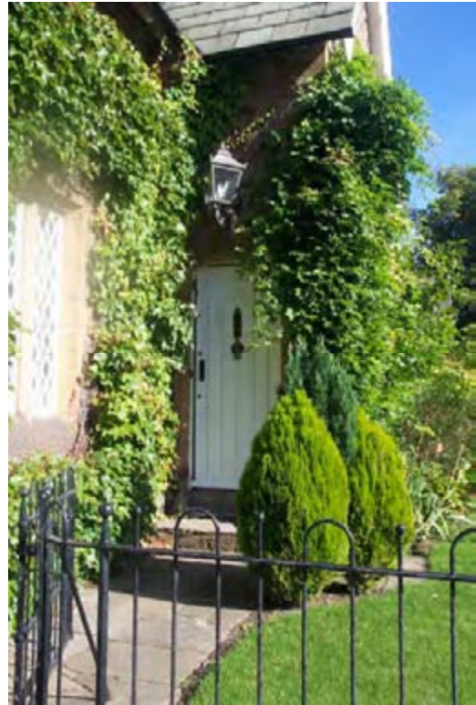
(8) Number 13 The Village a Grade II Listed Building occupying a prominent corner position in the village enhanced by well maintained landscaped elements.
