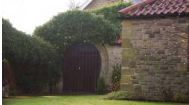
(21) The former Blacksmiths shop; now a private home and a valuable link to the village’s industrial past.
