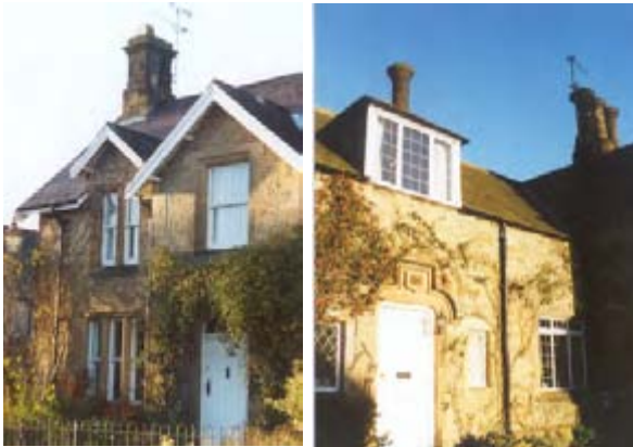
(23) Variation in window styles and detailing openings tend have flush stone lintels and projecting cills.
