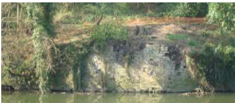
Image 185 Prebends Bridge and footings of the original timber structure
