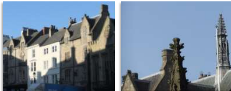
Image 152 Typical roof forms
