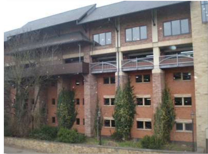
Image 163 Car park elevation overlooking the river
