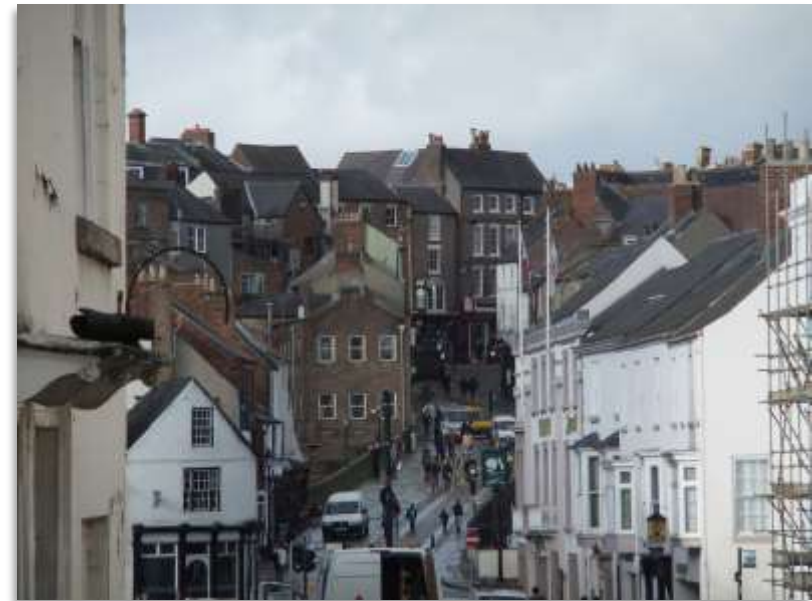
Image 129 Views of the roofscape from Elvet
