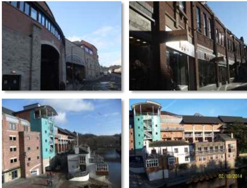
Image 160 Car park and service entrance, modest units, dominating stair tower
