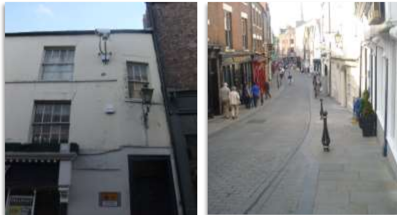
Image 138 Poorly maintained surface, modern interventions and general view
