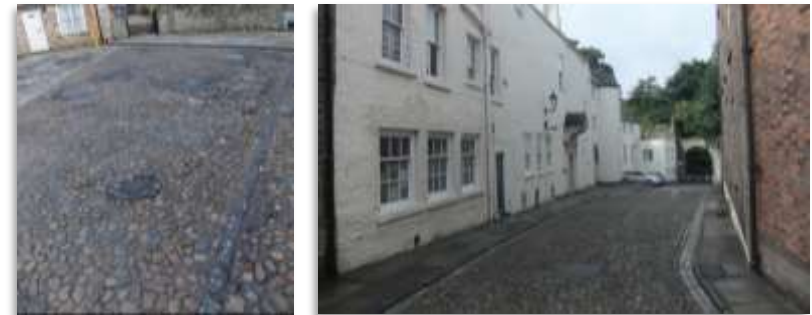
Image 119 Poor quality road markings and inappropriate repairs
