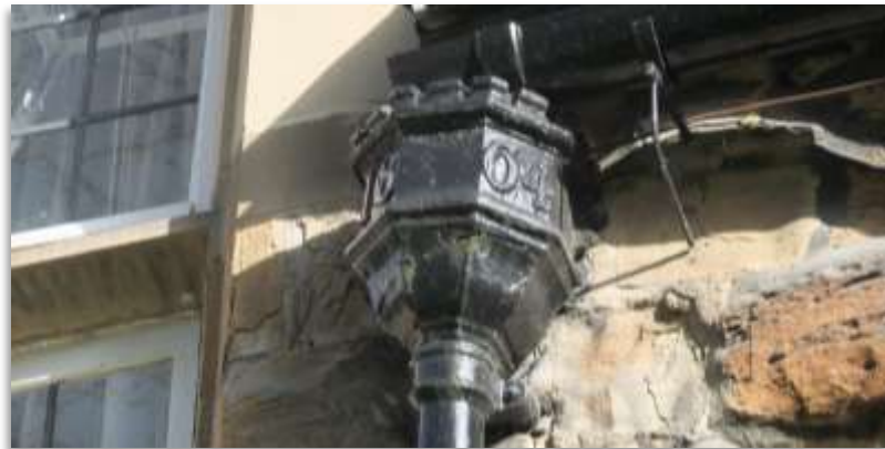
Image 107 Cast iron hopper heads and down pipes dominate
