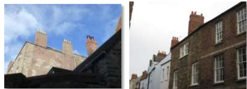
Image 106 Chimney stacks and varying roofscape
