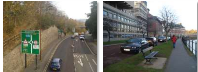
Image 25 A690 road cutting leading to Milburngate Bridge, riverbank and railway Viaduct (facing)
