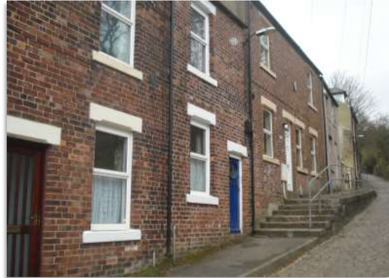
Image 59 Residential terraced properties at Sidegate
