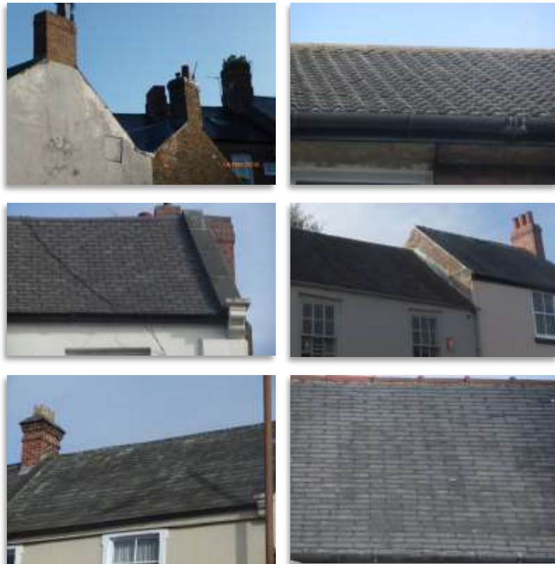
Image 118 Welsh slate dominates roof coverings
