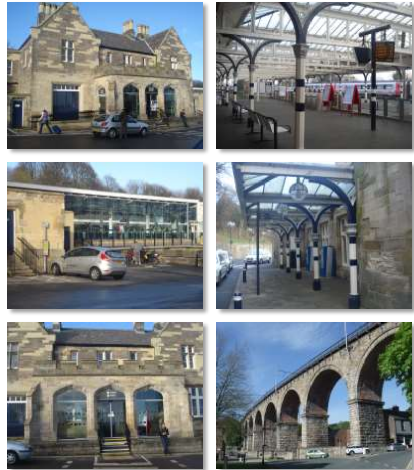
Image 36 The station complex and Viaduct
