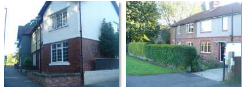
Image 10 Domestic properties along North Road
