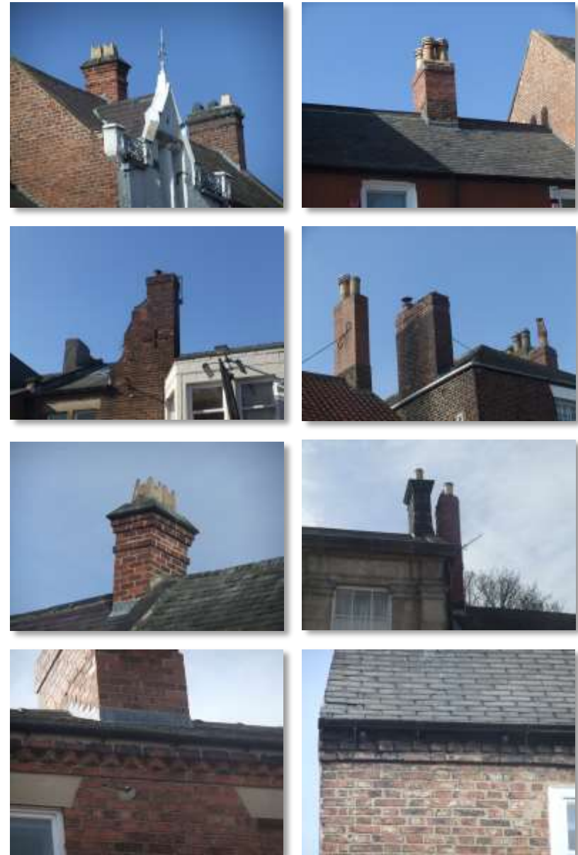
Image 119 Chimneys and roof details
