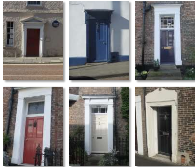
Image 122 Traditional timber doors
