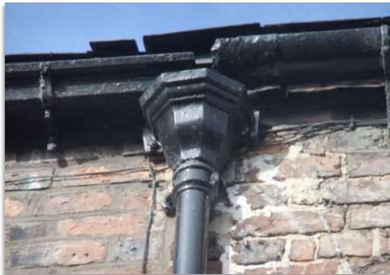
Image 120 Cast iron rainwater goods
