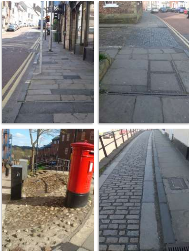
Image 135 Maintenance and clutter can be issues
