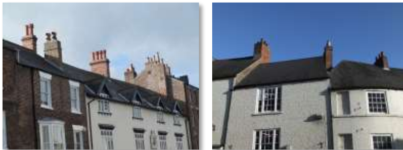
Image 36 Welsh slate is the predominant roofing material
