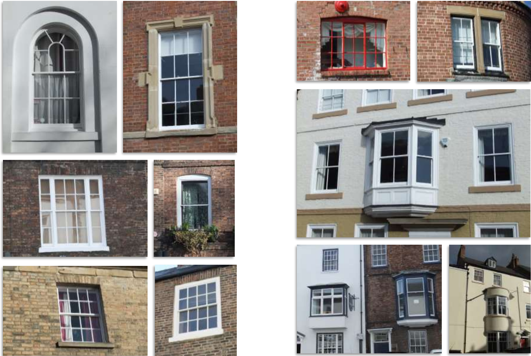
Image 39 Typical Elvet area windows
