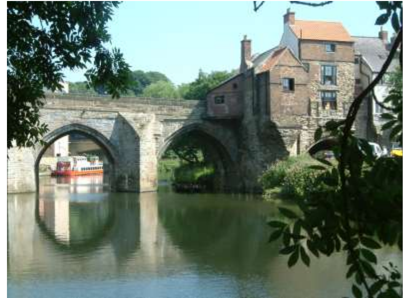
Image 20 Elvet Bridge to the rear of the eastern end
