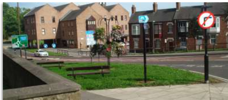
Image 50 Poor patching and clutter detract from the setting
