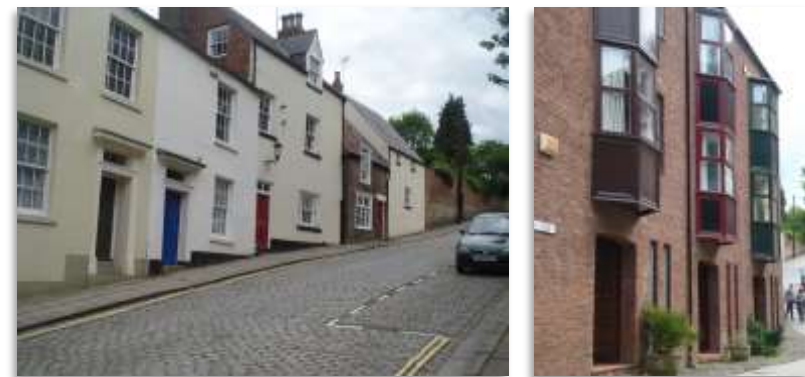
Image 72 South Street and Dunelm Court
