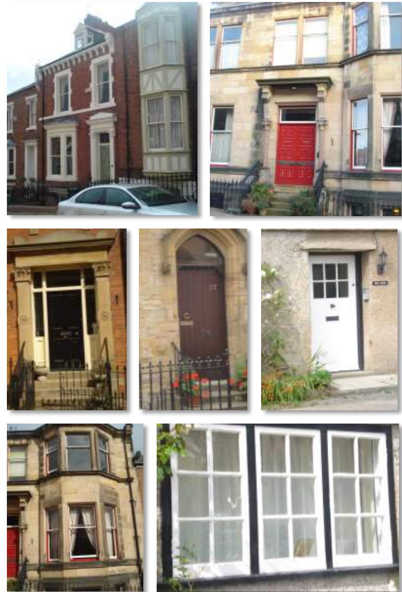
Image 12 High quality windows and doors
