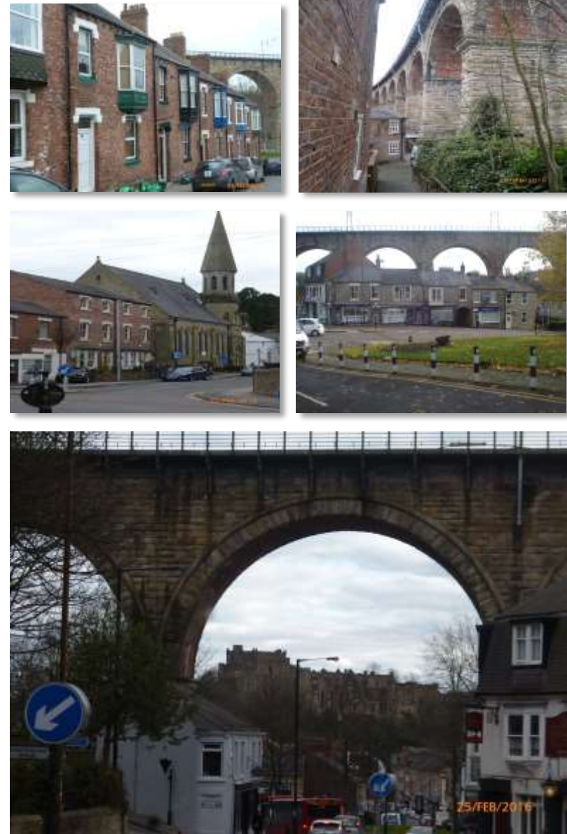
Image 4.6 Views around the viaduct
