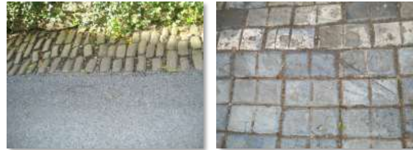
Image 21 Setts used to define pavements
