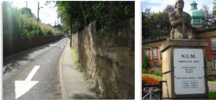
Image 35 Redhills Lane and the entrance to the Miners Hall
