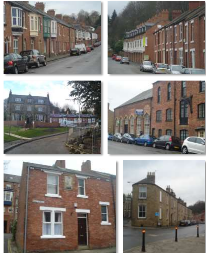
Image 104 Hawthorn Terrace, modern infill, Byland Lodge, former organ factory, May Street and Colpitts Hotel
