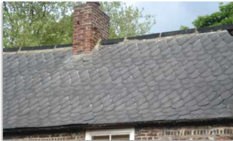
Image 138 Welsh slate is used widely
