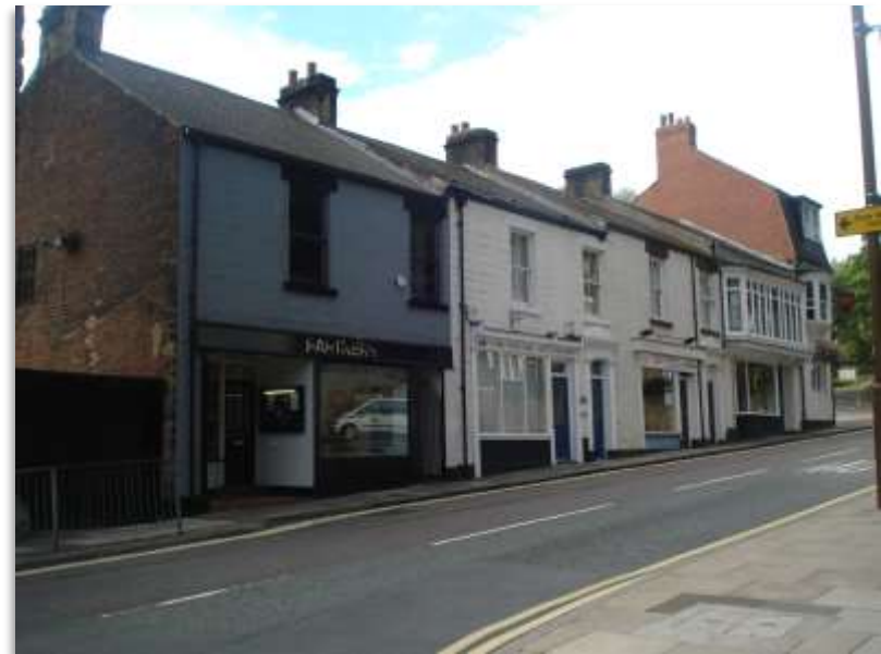
Image 29 Upper part of North Road beneath the Viaduct
