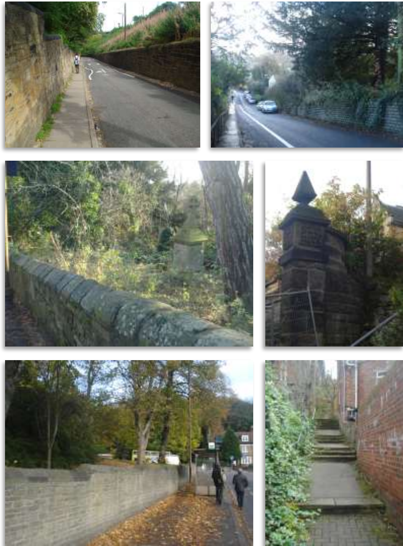
Image 44 Stone walls around larger properties
