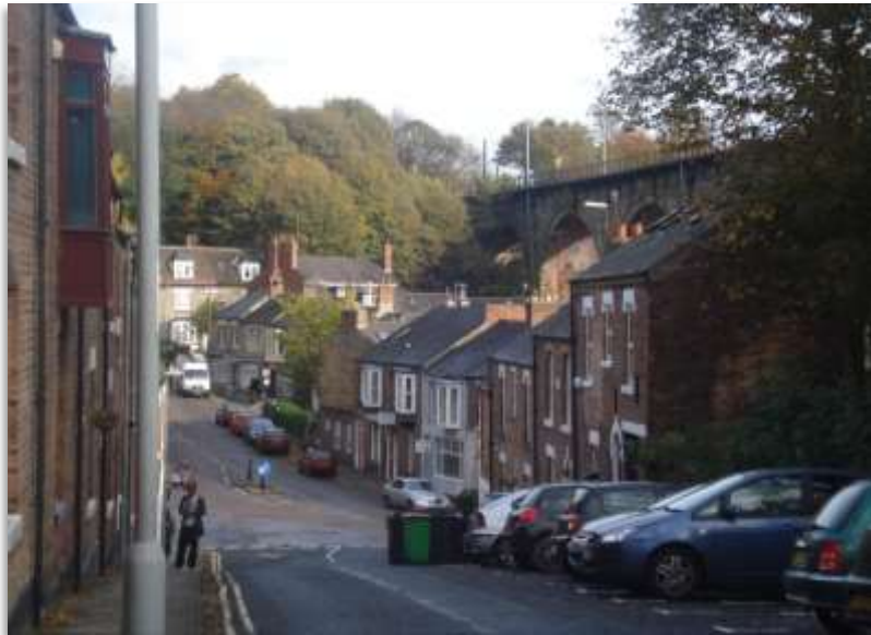
Image 47 Views along the terraces and around the Viaduct
