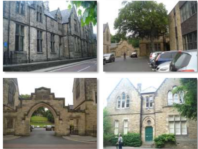
Image 126 Durham School, courtyard, entrance arch and Music Centre
