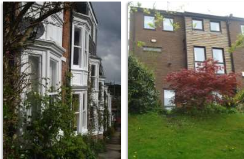
Image 139 Sash windows, elegant bays and modern top hung casement windows
