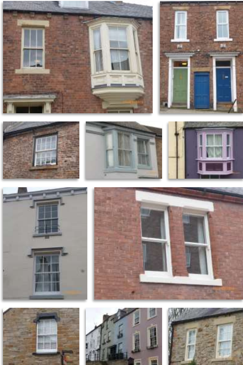
Image 81 (above and facing) Historic windows
