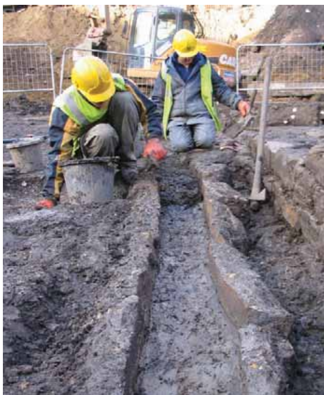
Figure 38 Excavation of drain features at Tuthill Stairs, Newcastle-upon-Tyne. These are characteristic of the site, which had been built on low-lying land reclaimed from the Tyne foreshore. © Tyne and Wear Museums
