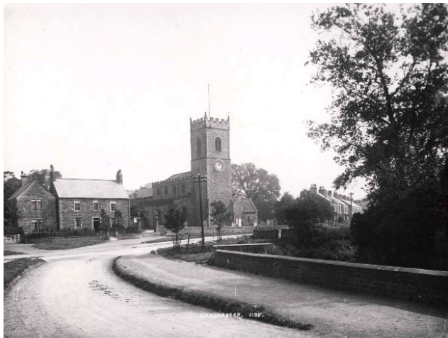
Before and after the by pass
