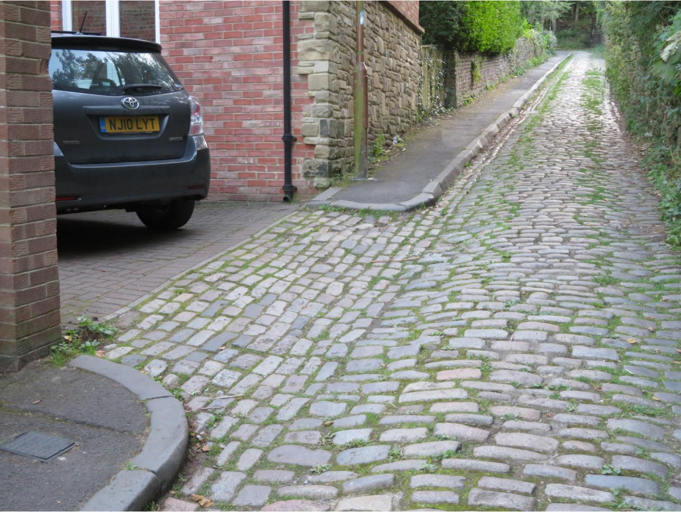
SNCF Appendix 20 Sidegate narrow, uneven, cobbled, unsuitable for limited mobility
