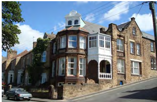
17 Aynsley Terrace – the most elaborately detailed townhouse. The level adornment was used to reflect wealth and prestige
