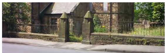
Iron railings outside St. Aidan's Church – rare survivors of railings within the conservation area
