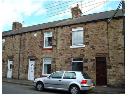
Overhead wires interrupt many views through the conservation area
