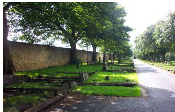
The stone wall that lines the east of the cemetery is a distinctive feature that provides a strong boundary to the space
