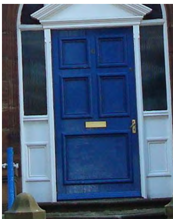
A multi-panelled timber door on Aynsley Terrace – a rare example of a surviving traditional door in the conservation area
