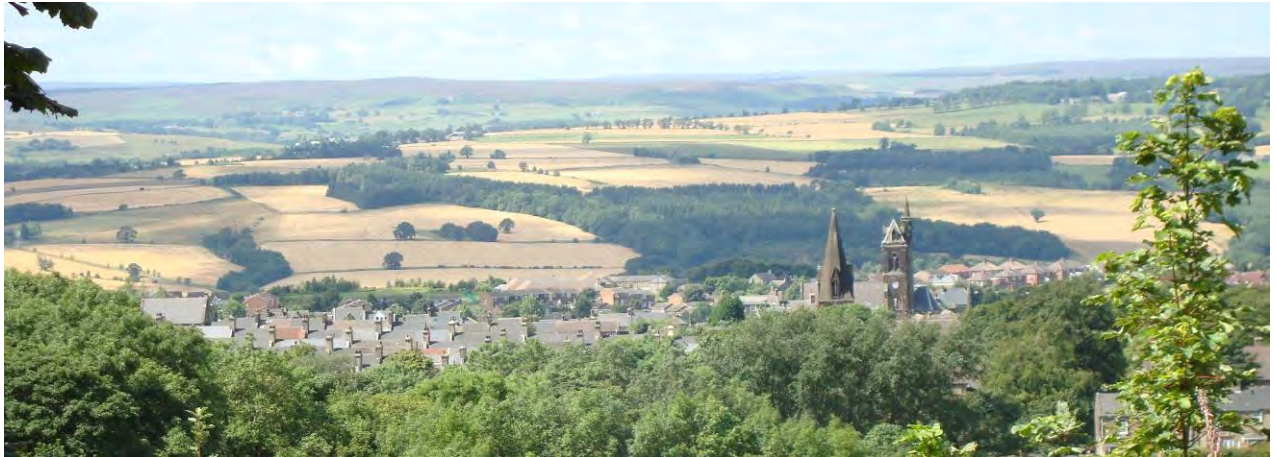
View over the roofs of Blackhill from Blue Heaps – the grey uniformity of the roofscape is a key characteristic of the place.
