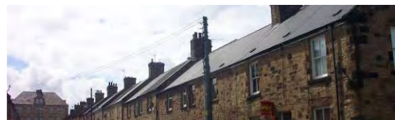
Welsh slate dominates the roofline, however modern materials have begun to undermine this uniformity
