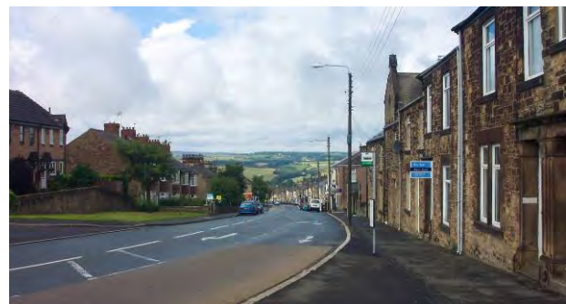
View along Durham Road towards the commercial core of Blackhill – visual connections with other parts of the settlement are important to the understanding of the conservation area
