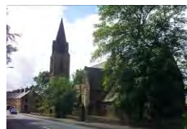
Church of St. Aidan Laburnum Avenue
