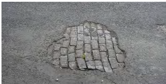
Granite setts are evident beneath the tarmacadum on Manse Road
