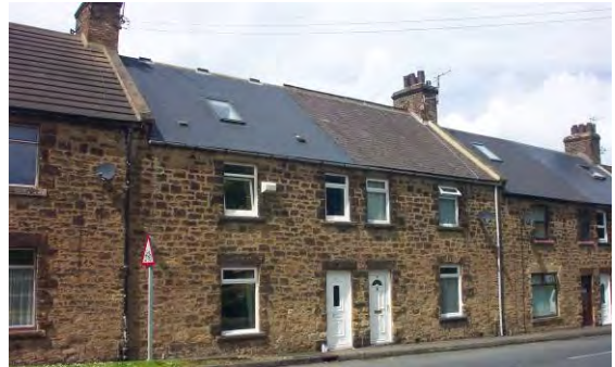
The uniformity of the roofscape of the conservation area is threatened by the use of modern roofing materials
