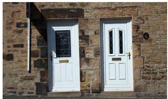
Quoins typically surround door and window openings and define the corners of the terraces.
