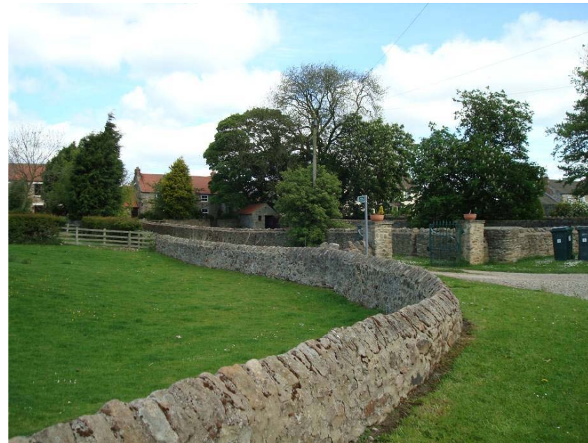
Stone boundary walls surrounding the garths are a significant feature of the village
