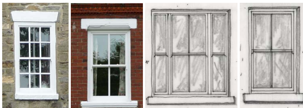
Plate 1. The sash window on the left is a style used prior to the 1860s. This was gradually replaced by the popular four or two light sash, made possible by advancements in glass technology. The two drawings are indicative of styles likely to be recommended in Cornforth. The tripartite sash window (second from right) is particularly useful for inserting into large window openings that may have once had a bay window, but where resources do not permit a new traditional bay. ‘Dummy’ sashes which open outwards are not appropriate.
