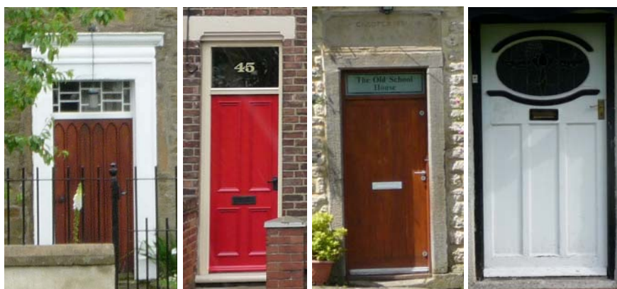
Plate 2. A range of traditional doors in Cornforth. Note the three on the left have no inbuilt lights. Hallways were lit by the overlight. However by the 1930s inbuilt door lights were being used (right). The four panel door (second from left) was the most common Victorian design. The door on the left is typical of the Gothic and Tudor styles revived in late Victorian times.
