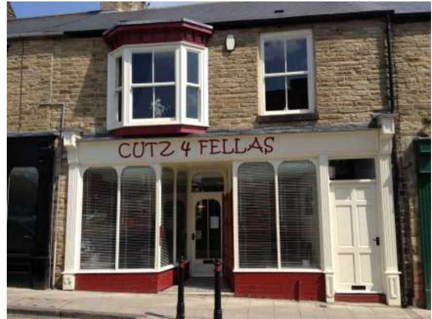
Traditional shop front on Hope Street
