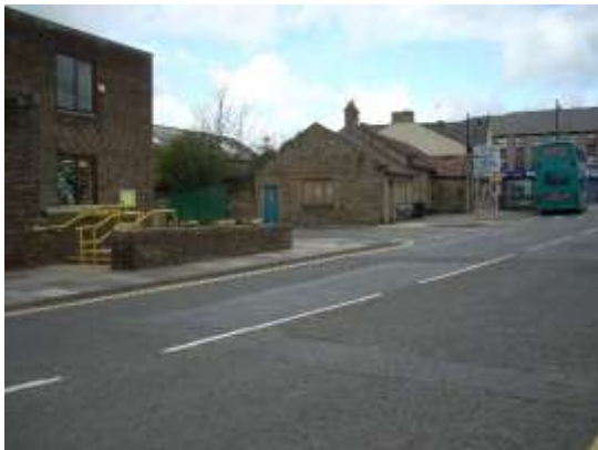
Former school building Elliott Street
