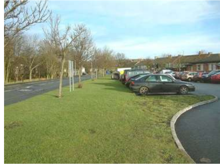
Crook Station site 2005
