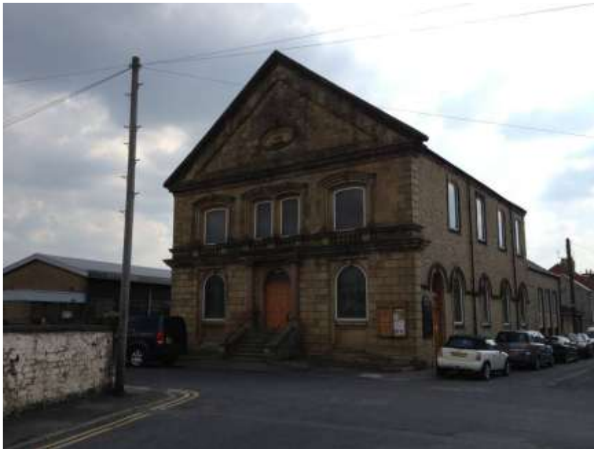
Central Methodist Church, Dawson Street
