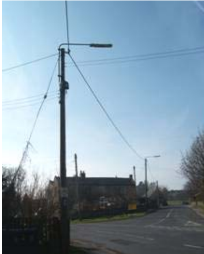
Hepple Hill. Street lights and overhead cables, east side of village.
