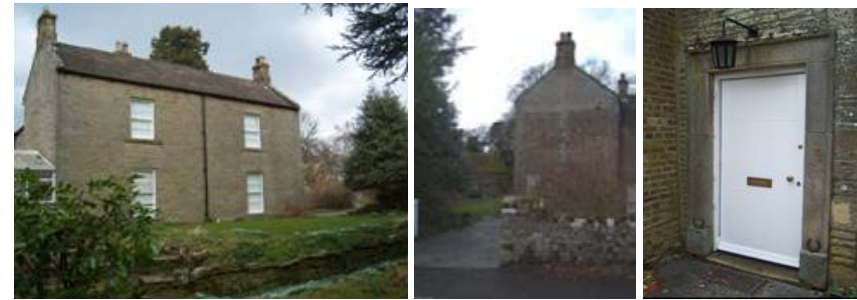
The Old Rectory from the churchyard to the south (above left). Left: doorway with datestone in east elevation. Above right: historic brickwork to east elevation.
