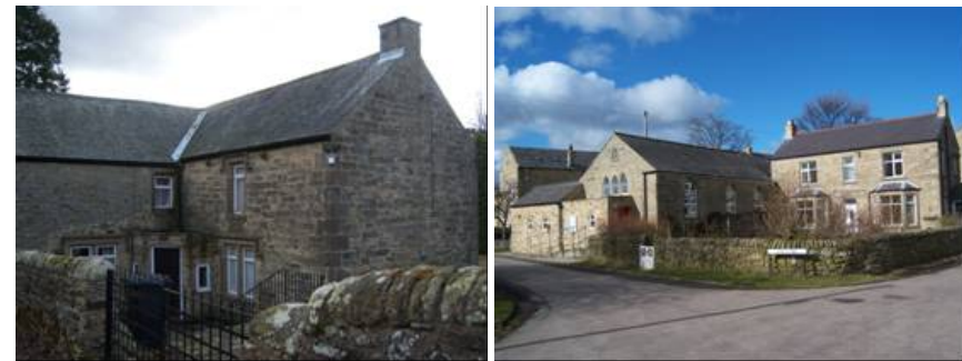
Left: Oldstead. Right: the old Wesleyan Chapel, now the village hall, and adjacent house.
