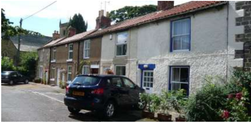
Church Row, a terrace of 18 th century cottages
