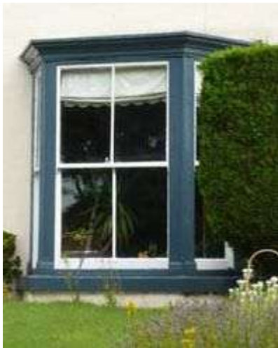
11 High Green late 19th, early 20th century splayed, canted bay with large panes with very simple framing and hood.
