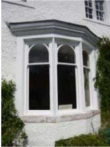
9 High Row, early 20th century canted bay windows with modillion decoration scrolls and interesting 'chink' decoration between sashes. An 'updated' Georgian design.
