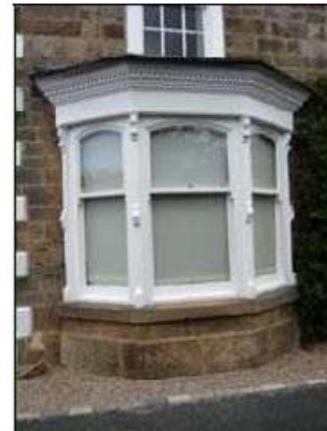
10 High Row, early 20th century canted bay windows with modillion decoration similar to no. 10 but much simpler framing including curving arched upper panes echoing art deco.
