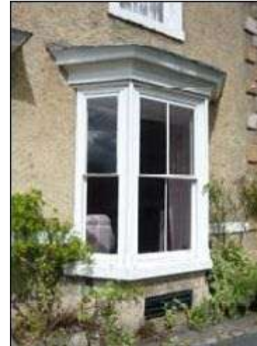
8 High Row, mid to late 19th century flanking, square, canted bays, quite simple in design with large rectangular panes and thin, roll moulding on the framing and canopy.
