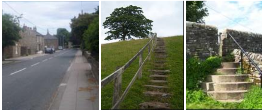
Concrete flags and stone steps
