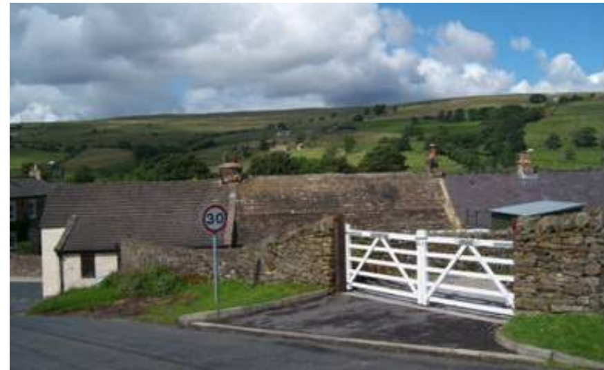
Contrasting roofs: modern artificial slates (left), traditional stone flags (centre) and Welsh slate (right on Front Street).
