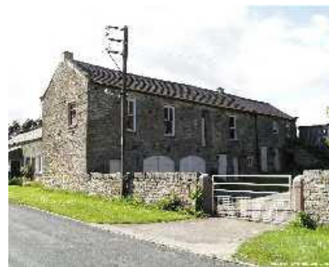
Outbuildings west of The Grove
