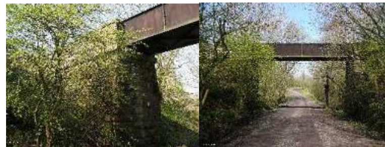
Aqueduct abutment Aqueduct trough
