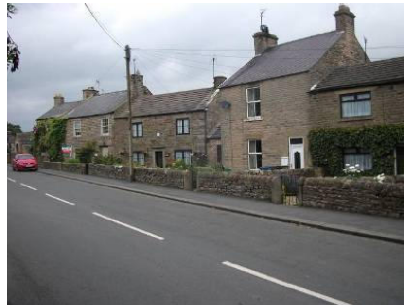
Stone boundary walls and inappropriate replacement windows
