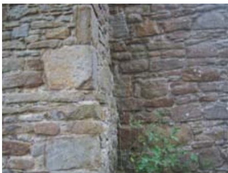
In situ medieval masonry at the Grange ruins.
