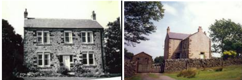
Sunny Bank. Top left: Front elevation, 1950s. (Source: M Sobo archive) rear elevations, 1993 (Photos: M Sobo).
