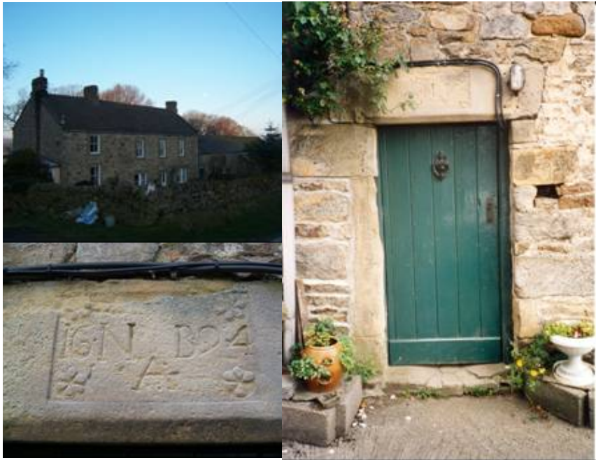
Grange Farmhouse, late 17th century doorway with datestone above (photographed in 1999 by M Sobo). Detail of datestone in 2008, showing erosion
