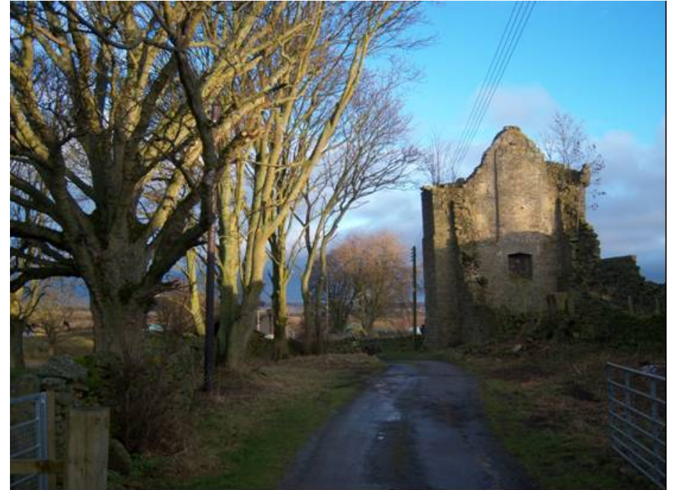
The Grange ruins from the road, showing the west (internal) face of the east gable of the east block.
