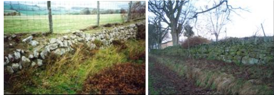
Left: Roadside wall with overlying fence on the line of the medieval park boundary north-west of Lane Head (outside the conservation area) – walls of this form may originally have been hedgebanks and may well have medieval origins. Right: Roadside wall incorporating large boulders, south of Sunny Bank.
