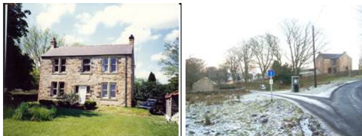
Left: Front elevation right: the house occupies a key location above the junction of the Muggleswick road (the other building is the Old Smithy).
