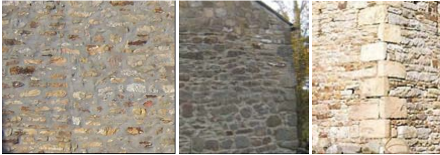
Examples of historic masonry within the conservation area.
