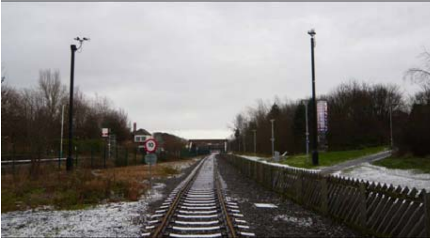
View east down the track towards the Shildon station signal box and the Spout Lane bridge at the east end of the site
