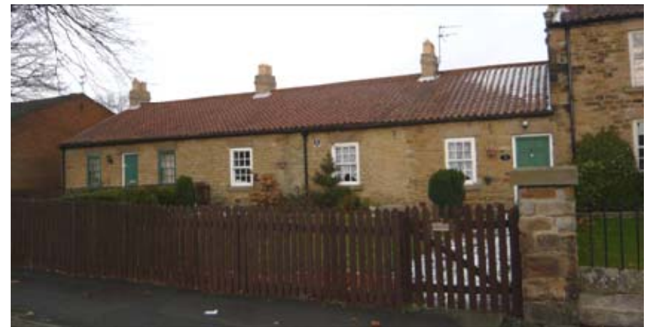
Worker's cottages adjacent to Hackworth's house; these are the earliest examples of worker's housing on the site
