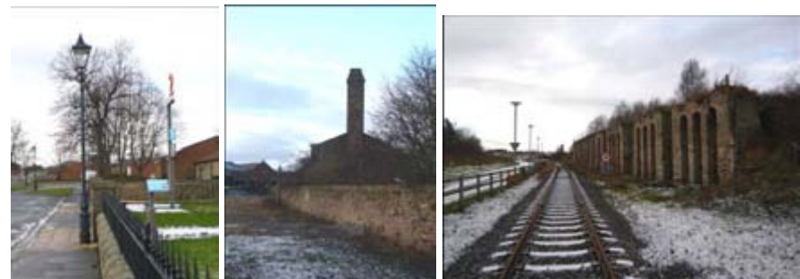
One of Shildon's gas lamp posts with adjacent railings in front of Hackworth's house. The Grade II listed wall south of the engine house and sections of surviving track add context and depth to the area's surviving buildings, and were repaired in 2008.
