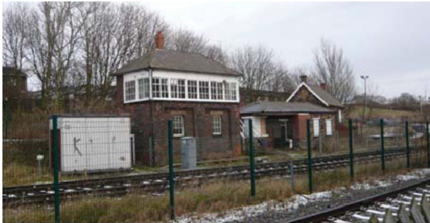
Listed signal box and associated buildings, although currently outside the conservation area these buildings constitute a prominent group which can be seen from a number of vantage points
