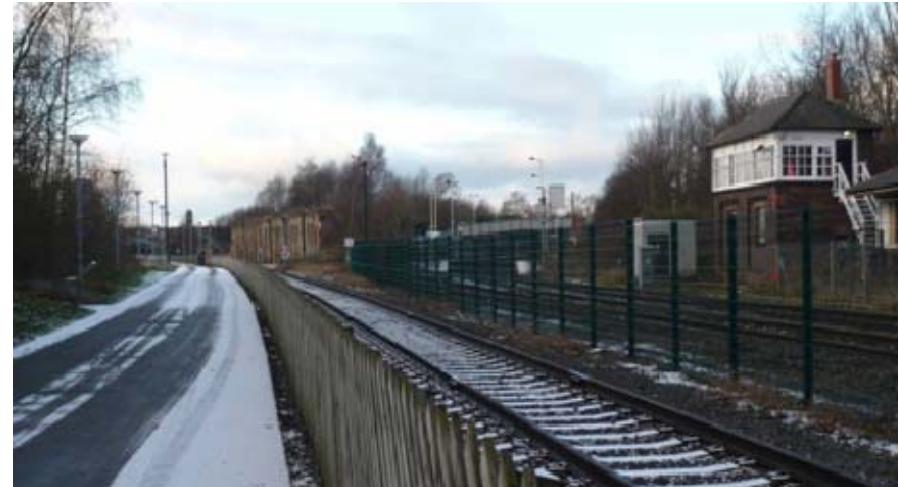
View west from just underneath the railway bridge at the eastern end of the area. This is the primary view for visitors approaching from Locomotion.
