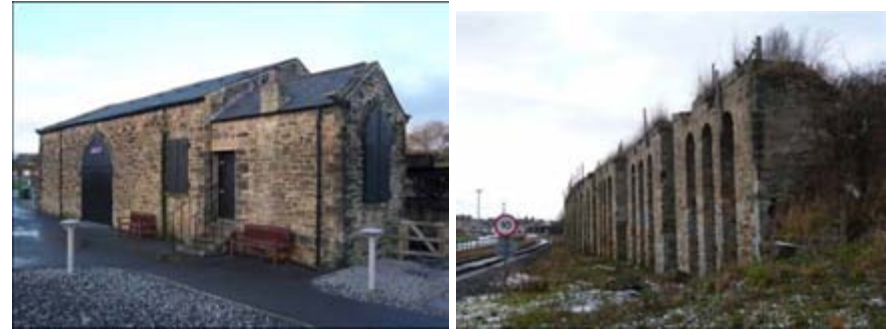
The goods shed and coal drops; both date to a second phase of development surrounding the Soho Works
