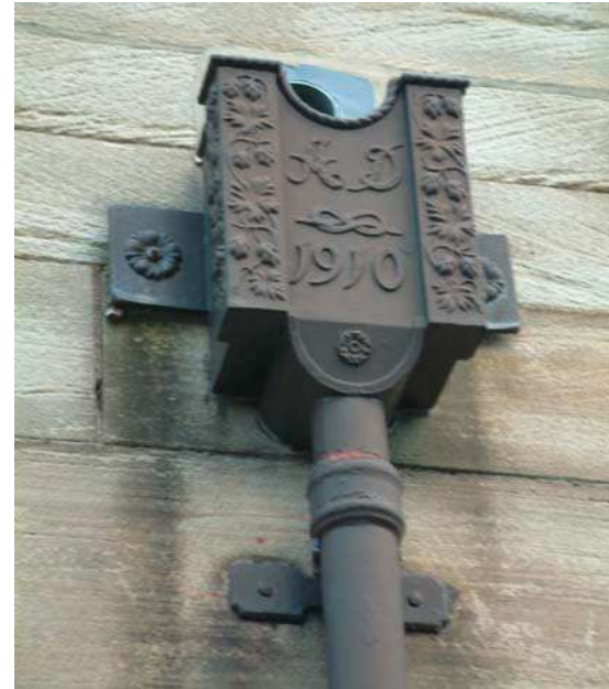
Cast iron rainwater goods on the King James I School.
