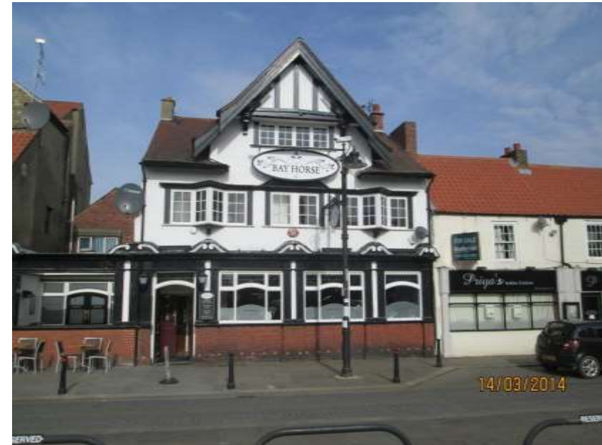
Bay Horse Public House, Fore Bondgate
