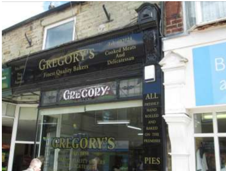
Historic timber mouldings and timber detailing
