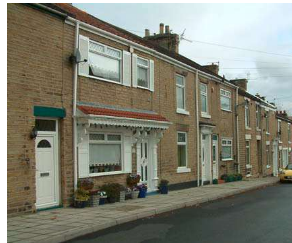
Replacement windows and doors on Russell Street.
