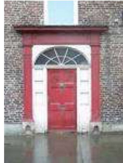
Traditional door detailing Market Place
