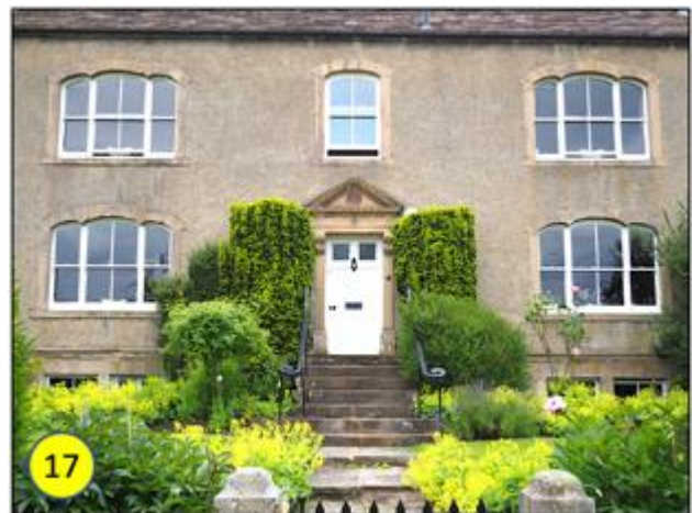
Figure 17: Showing decorative stonework and detailing to door and windows
