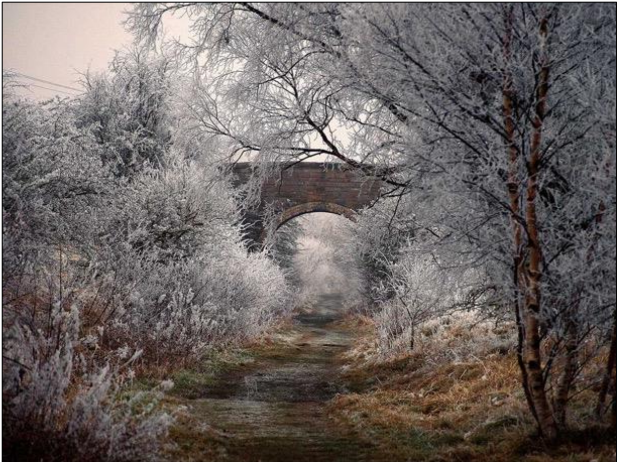
LVHA14: Tees Railway Path – former railway line and bridge in wintertime
