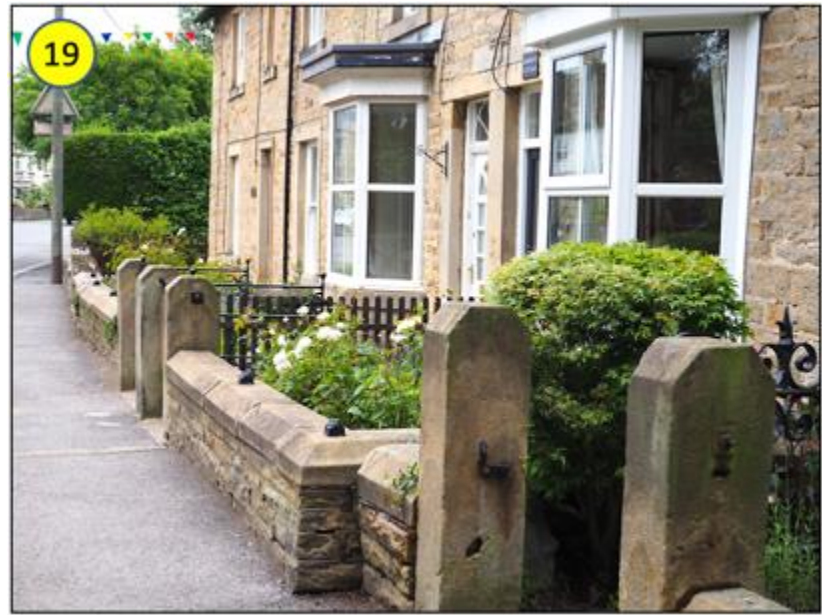
Figure 19: Traditional low stone walls, with dressed copings, originally topped with iron railings (now lost)
