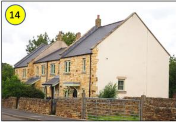
Figure 14: Modern development successfully combining stone on principal elevation with rendered gable
