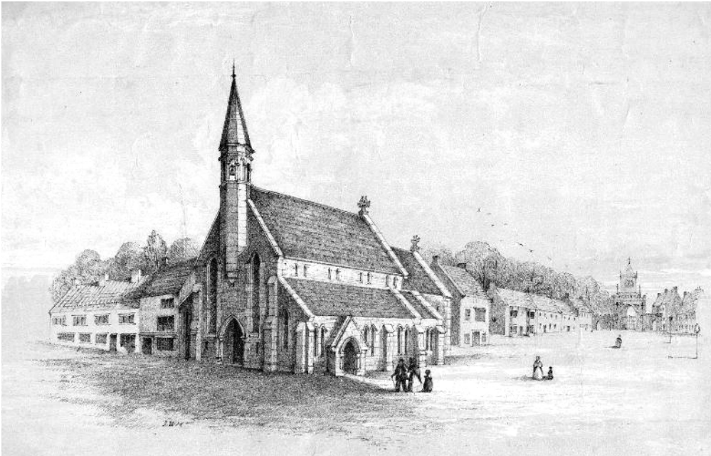
St Anne's Church following rebuilding
