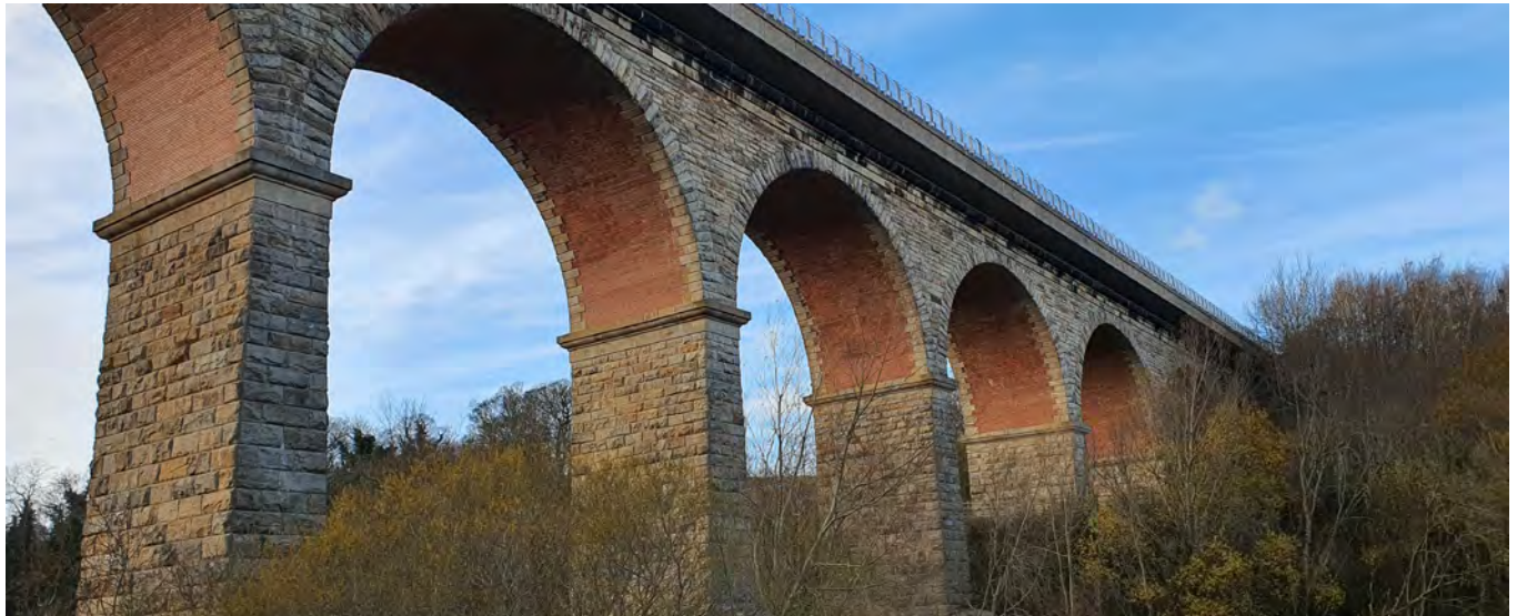
Newton Cap Viaduct from The Batts
