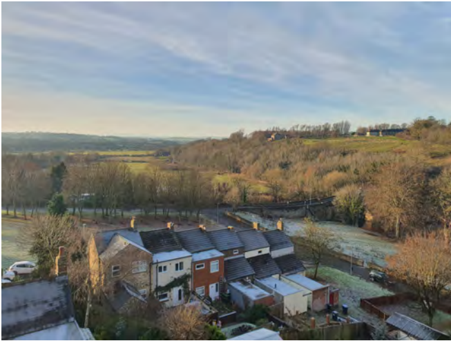
View 01a: View east from the viaduct towards Newton Cap Bridge
