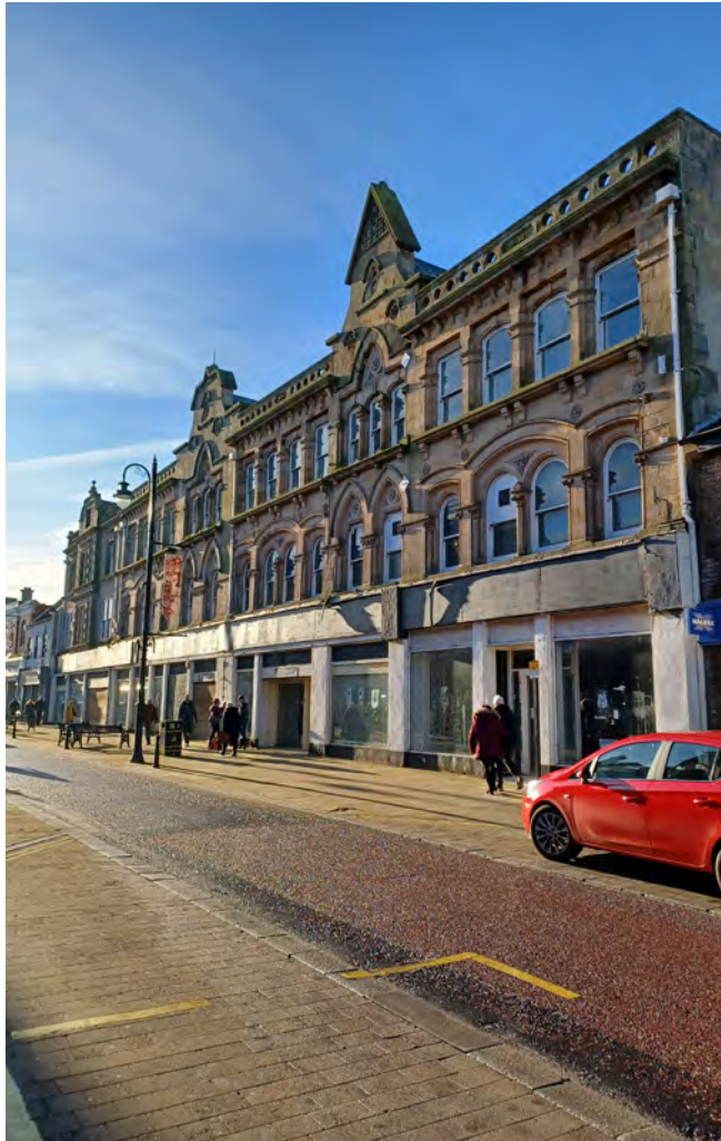
Now vacant former Co-operative store on Newgate Street
