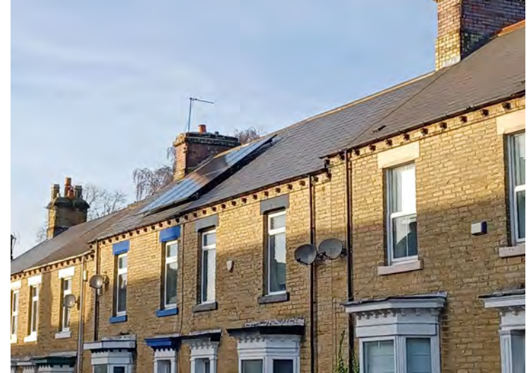
Satellite dishes and PV panels in the character area
