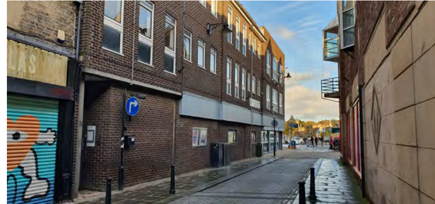
Modern intrusions on Fore Bondgate
