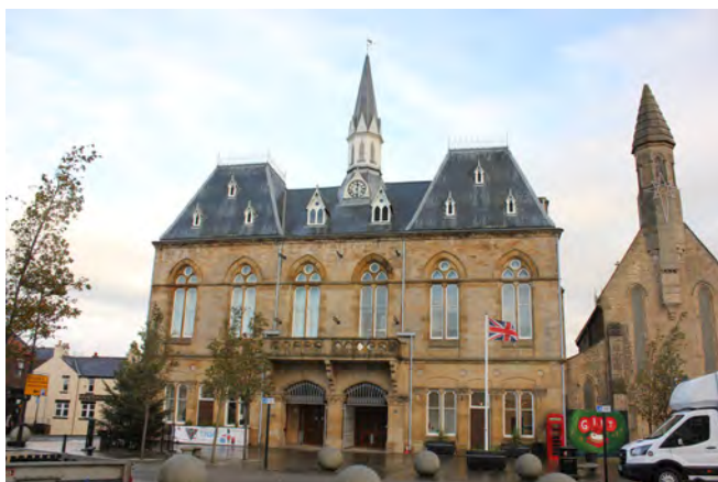
The Town Hall, now a library and community arts hub
