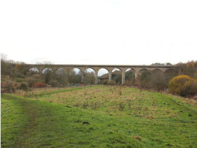
View 02: Newton Cap Railway Viaduct from The Batts
