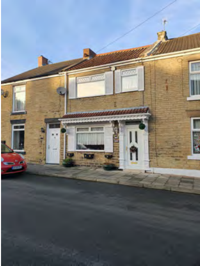
Loss of original windows and openings and a desire for individuality has made this house unrecognisable as a Victorian worker's cottage
