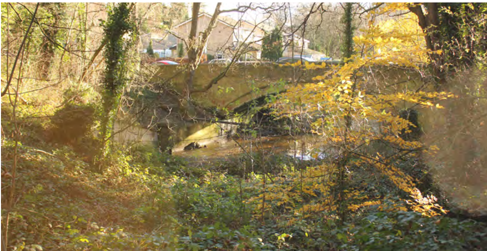
Bridge over the river Gaunless, Durham Chare
