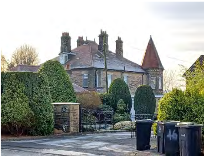
No.58 Etherley Lane
