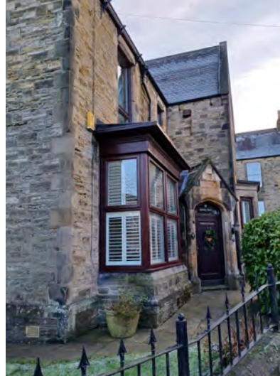
UPVC windows are common within the conservation area
