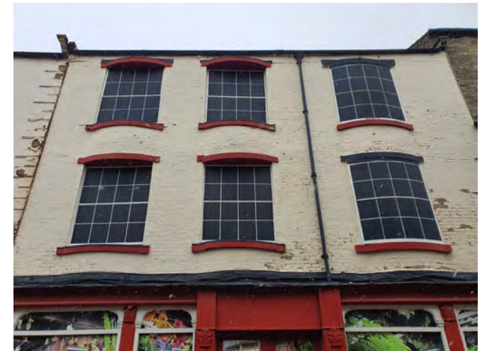
Remains of Late Georgian shallow bow bay windows in Fore Bondgate
