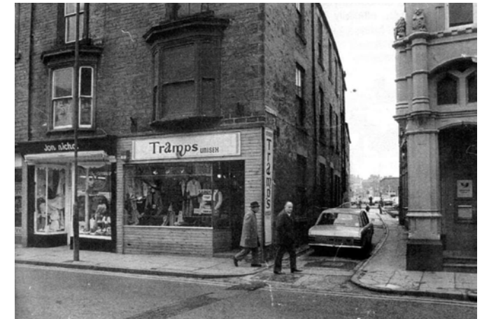
William Street before the construction of the Newgate Street Shopping Centre
