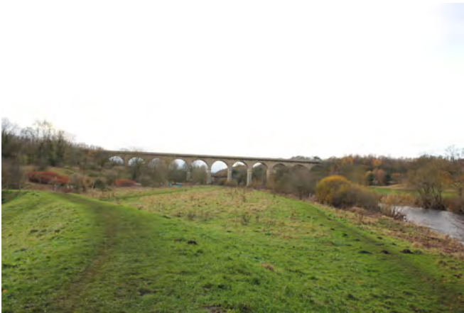
Riverside walk along the Wear, looking west at the Newton Cap Viaduct
