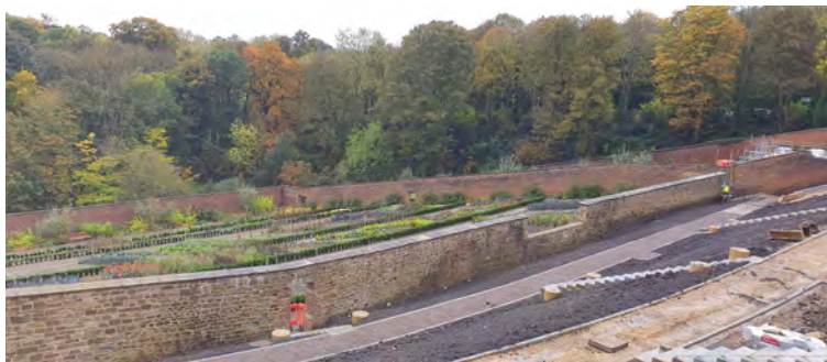
Walled garden undergoing restoration
