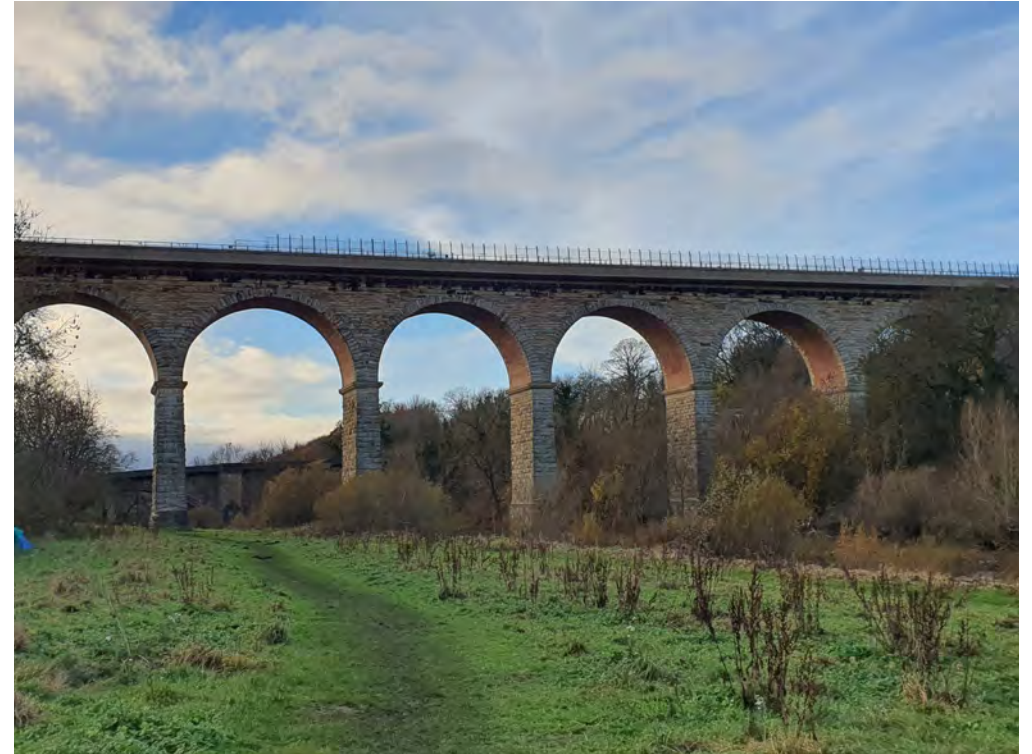
Newton Cap Viaduct from The Batts
