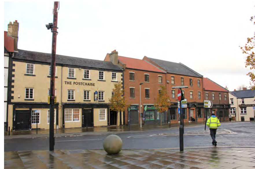
Vacant buildings on Market Place
