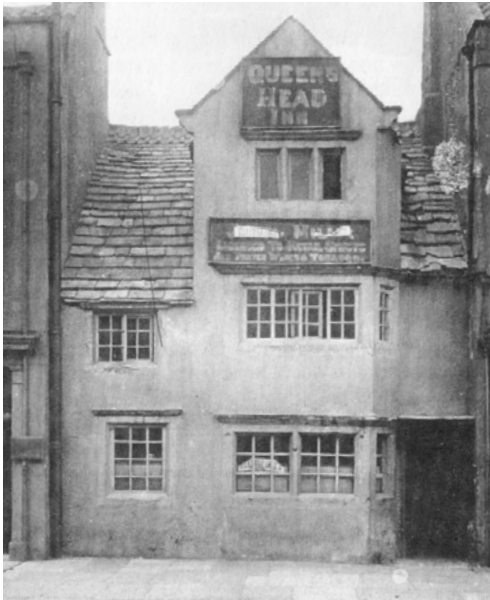
Queen's Head before demolition c.1898
