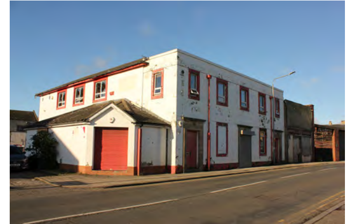
Derelict building on Kingsway
