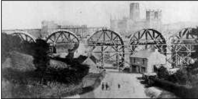
Fig 30 , construction of Durham Railway Viaduct 1857, County Records Office
