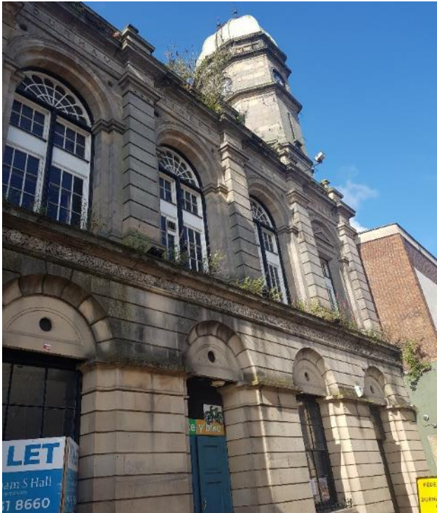
Fig 77 examples of different buildings at risk, the former Miners Hall North Road, South Street Mill building on the riverbanks, the redundant Edwardian outbuildings at Mount Joy Farm, and former public swimming baths at Elvet Riverside.
