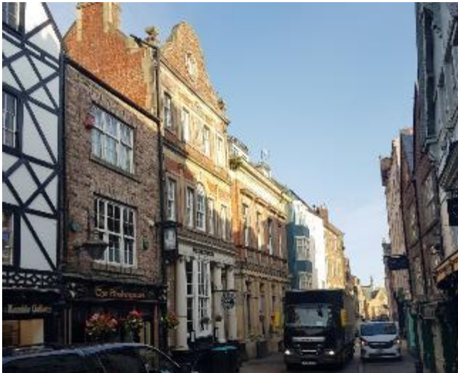
Fig 20, view of the different architectural styles to the historic buildings along Sadler Street.
