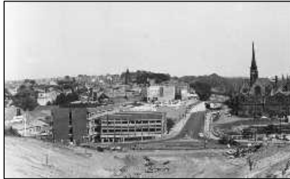
Fig 32 , construction of the through road and bridge 1970-80, Durham County Records Office.
