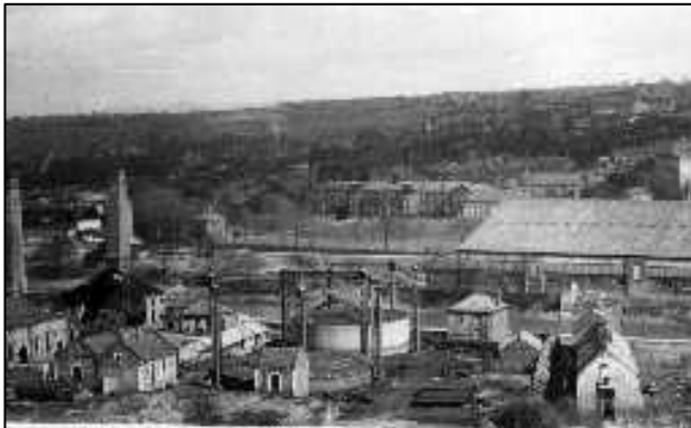
Fig 39, view of the riverside 1950s-75, Durham County Records Office (Ref.DR00805), showing the gas works and ice rink. The far side of the river is now the site Freemans Reach, Wearside House and the University Business School.
