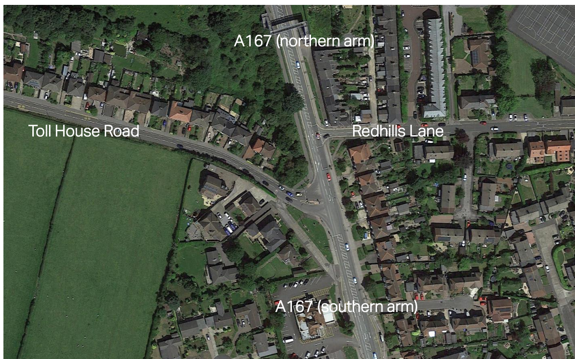
Figure 2-2: Toll House Road Junction
