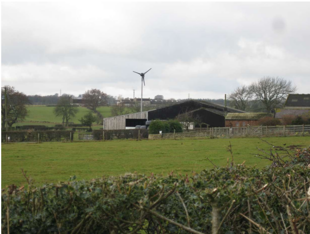
Figure 17 Small turbine (18m) at Bolton Hill
