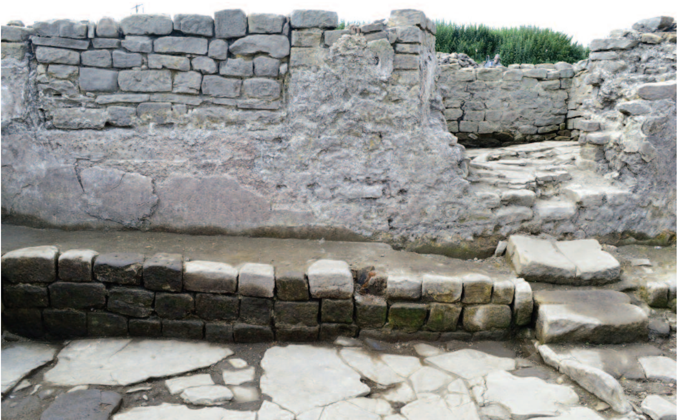
11. Bath-building, west wall of apodyterium showing blocked-up window embrasure to left and cut-down window embrasure with inserted steps to right.
