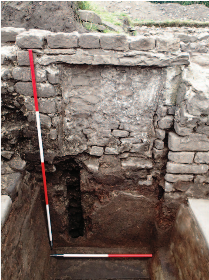
21. West wall of plunge-bath showing blocked-up window and damage resulting from the robbing-out in antiquity of a lead water pipe (?).
